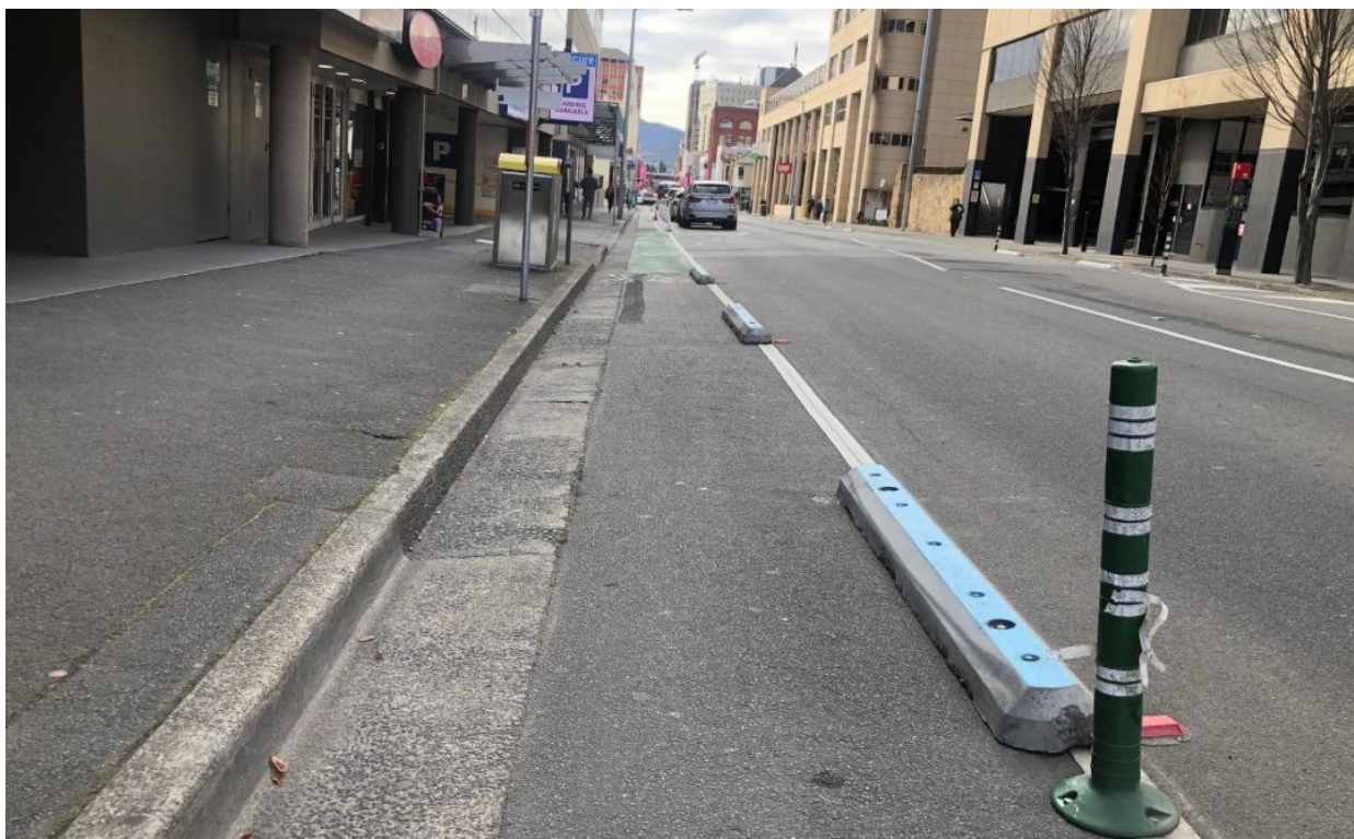
Figure 9 Concrete Wheel Stop Separators
